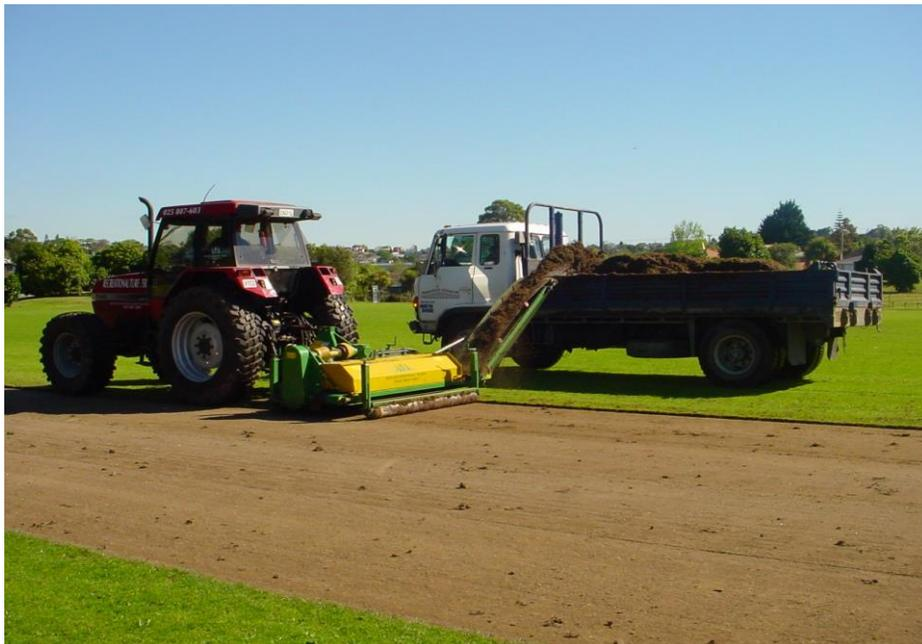
**Use of field topmaker to blade off the turf surface.**
